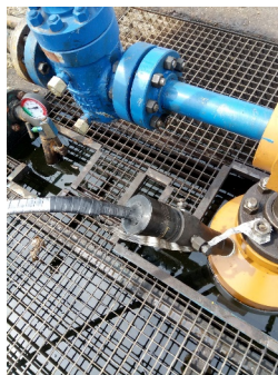
Cable packoff hardware can be used with a wellhead adapter (left), or it can be run through the annulus (right).
